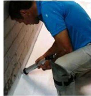
Wet Area Waterproofing
