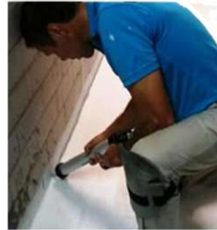
Wet Area Waterproofing
